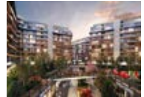
Lens İstanbul Property type: Residential Developer: Lens Construction Number of residences: 982
