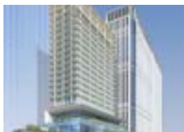
Shin-Tekko Building Property type: Residential Developer: Oakwood, Mitsubishi-Jisho Number of residences: 54
