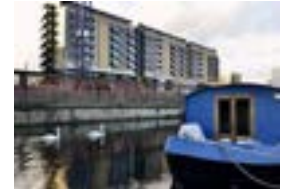
Suttons Wharf North Property type: Residential Developer: Hollybrook Number of residences: 450
