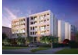
Axial Apartments Property type: Residential Developer: Colin Stewart Architects and Bloc builders
